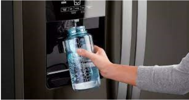
FRIDGE COLD WATER LINE
